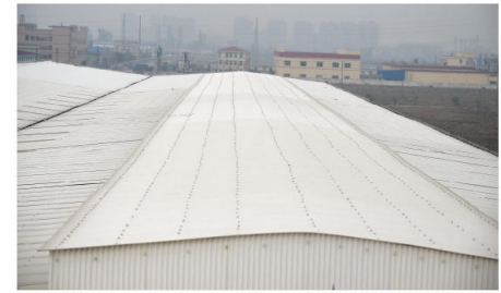
Gaoyao Plastic plant(project date:2015)
