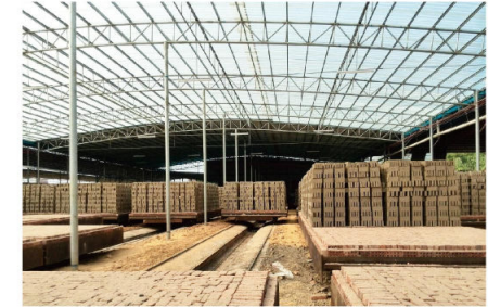
Yangchun Air field of Brick Yard(project date:2015)
