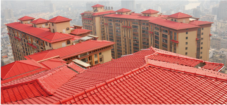
GuangXi Junxin international building(project date:2016)
