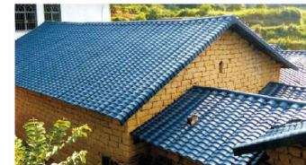
Zhejiang Houses renovation ( project date :2015 )
