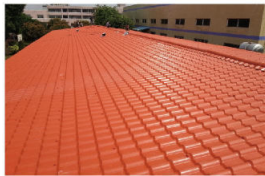
Fujian Living Quarters(project date:2013)
