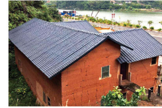
Hunan Houses renovation ( project date :2015 )
