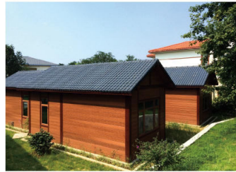
Qingyuan renovation project(project date:2014)
