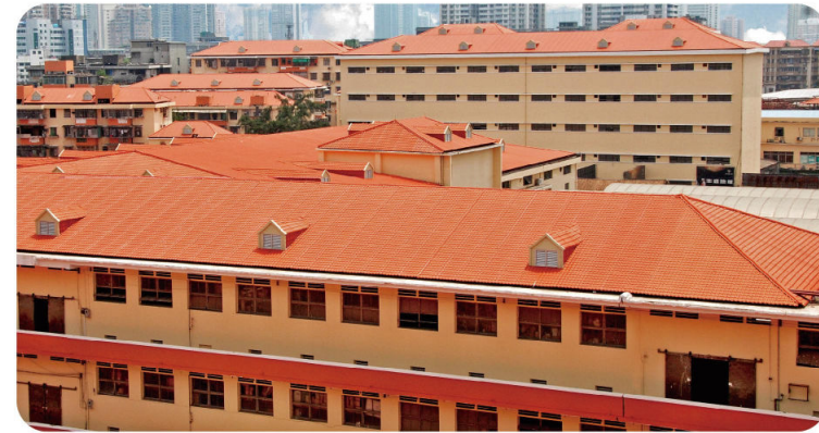
Guangzhou flat-to-sloping roof project(project date:2015)
