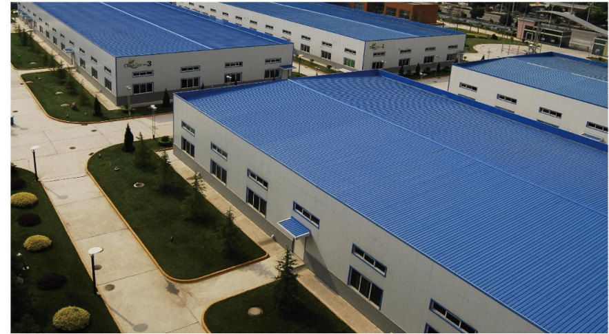
ZheJiang Steel Plant(project date:2014)
