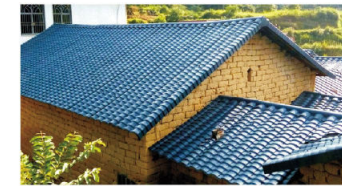
Zhejiang Houses renovation ( project date :2015 )
