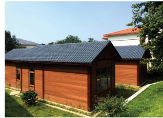
Qingyuan renovation project(project date:2014)
