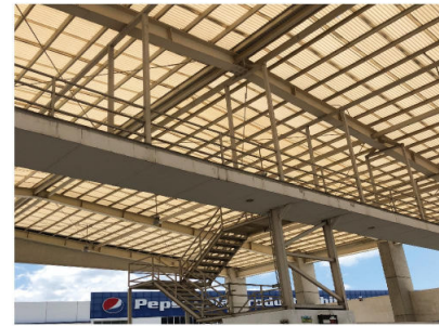
Pepsi Cola factory abroad(project date:2017)
