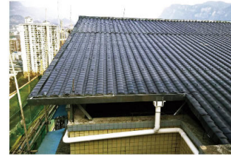
Guizhou Sinan County New rural reconstruction project ( project date :2017 )
