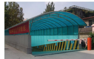
Cell Carport Entrance(project date:2015)
