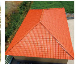
Jiangxi Residential Renovation Project (project date:2013)
