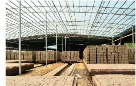
Yangchun Air field of Brick Yard(project date:2015)
