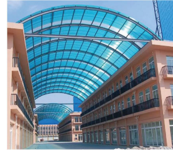
Factory waterproof sunshade(project date:2015)
